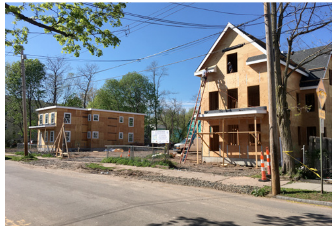
Construction along Thompson Street.
