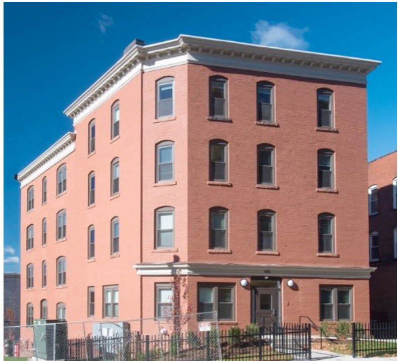
445 Zion Street – Before and After. Source: Mutual Housing Association of Greater Hartford.
