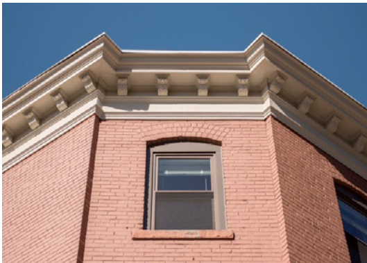
445 Zion Street – Architectural detail. Source: Mutual Housing Association of Greater Hartford.
